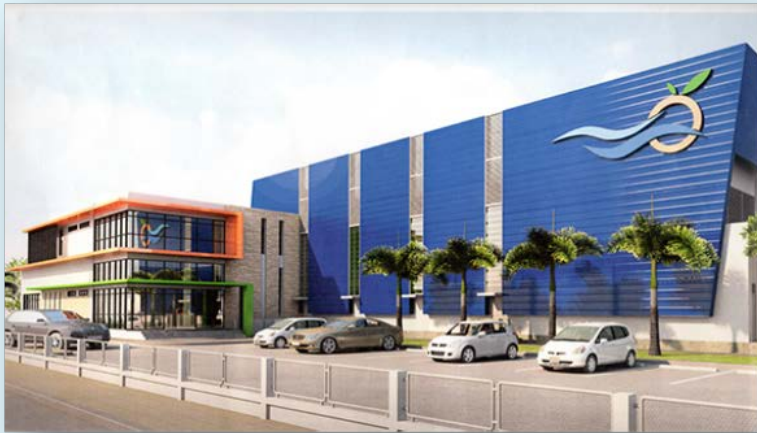
Food Innovative Service Plant (FISP)
